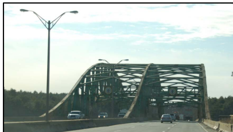
Whittier Bridge looking south
